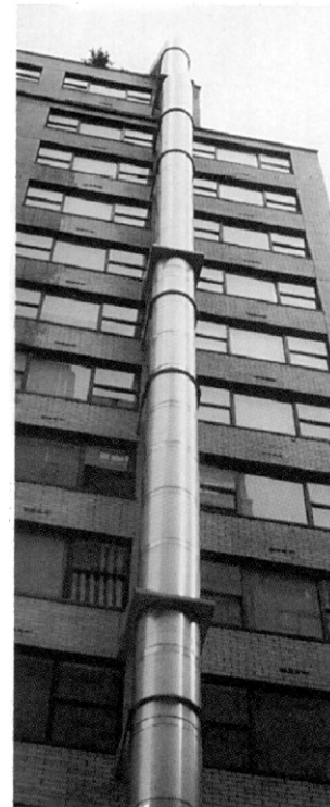
With proper support, Schebler chimney components can be used to make stacks of virtually any height. The stack shown here uses wall supports and wall guides to support the chimney along the building structure.
